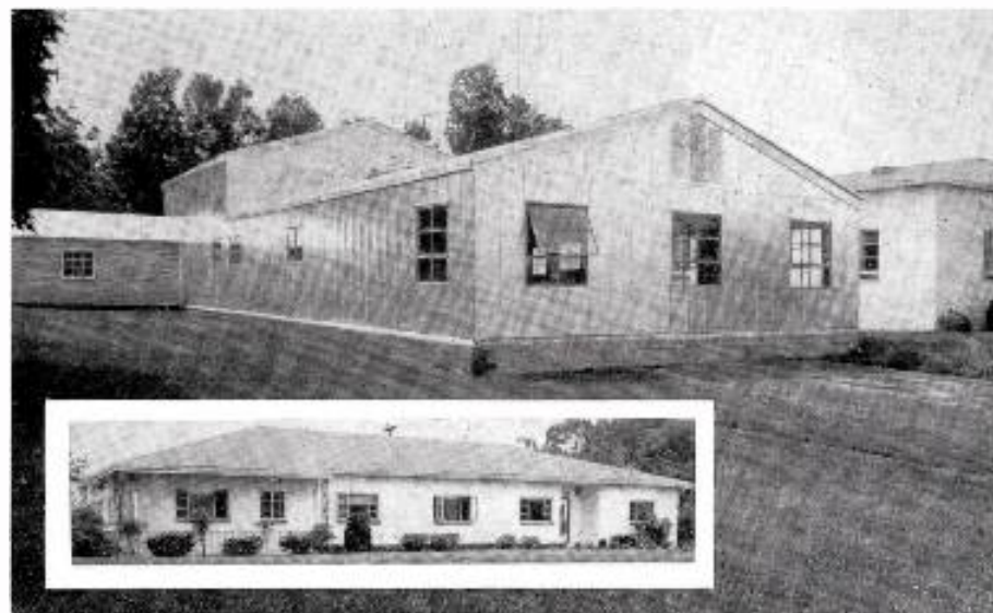
FROM the office end, WSVa-TV's new metal studio-office building looks like this. At extreme left is the old metal garage used for storage. At rear is the studio end of the building, with higher ceilings to accommodate props and lights. Inset shows the original WSVa plant, which includes both radio and tv executive offices.
